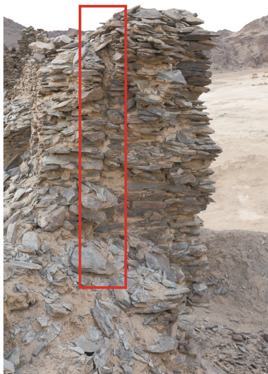
Figure 4. Absence of masonry connection facing along the northeastern wall. Photo: D. Fedorova
